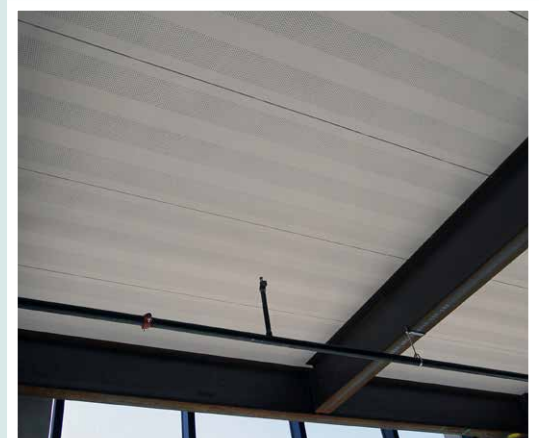
Smooth Series Cellular Deck provides a clean beam-to-pan rivet attachment.
